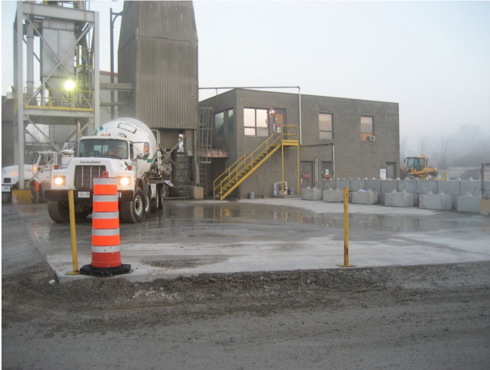
Figure 6.1 Paving at a ready mixed concrete plant in Quebec.
