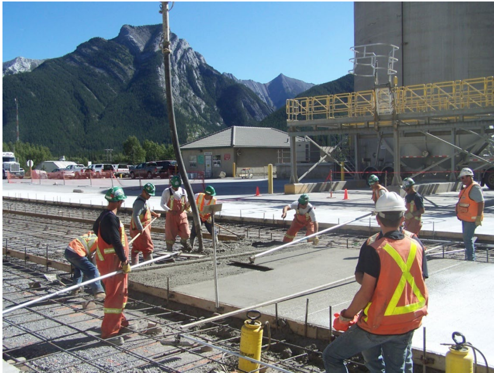
Figure 6.2 Paving at a cement plant in Alberta.
